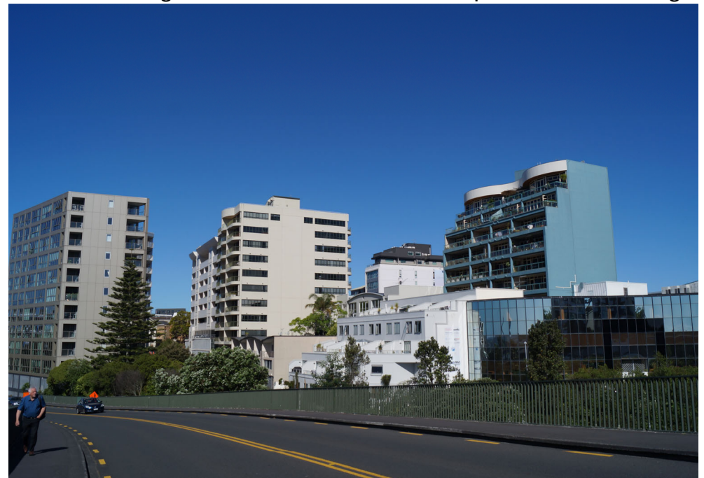
View of Avoka Apartments from Hopetoun Street Bridge
